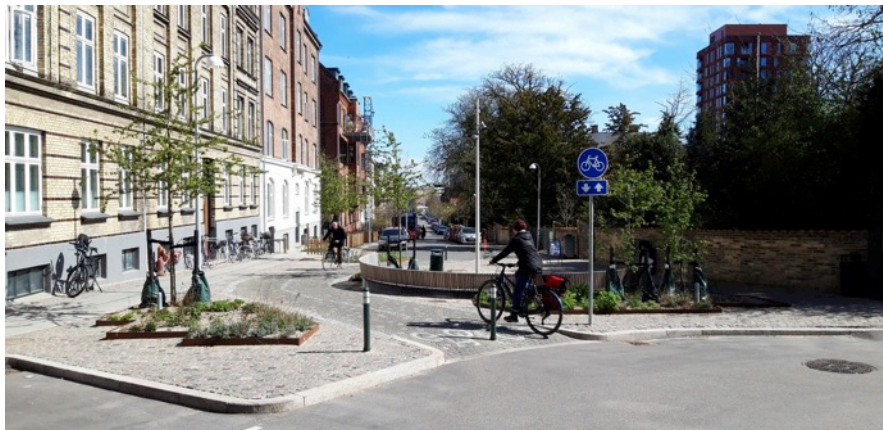
Fig. 2: This junction in Copenhagen has been structurally reconfigured to allow pedestrian and bicycle traffic to continue and motor vehicle traffic to turn right. The areas acquired are used for recreation. (Photo: H. Hagedorn)
